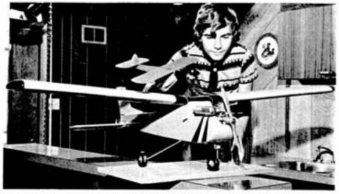
Filteen-year-old Mark Quellet compares the targest and the smallest in the family's fleet of forty gas powered flying model aircraft. Motor on the small plane packs 0.1 hp, revs at 20,000 rpm and costs about \$10. Motor on the large plane has a 1.5 hp punch, revs at 10,000 rpm and is worth \$70.
