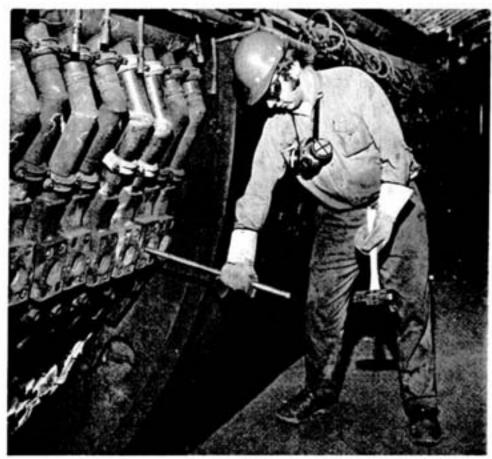
A familiar scene to the many old timers who for many years punched converter tuyeres-hand punching with puncher Mike Brujic wielding the hammer. With the development of the "Gaspe Puncher" this scene and the need for hand punching will be relegated to the past.
