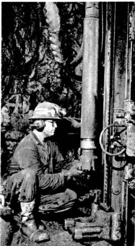
Driller Jack Wallgren checks the button bit on his "COP 6" down-the-hole drill. That four-foot section of drill rod or tube, up to the first joint, contains the impact mechanism or drill that is always down the hole, the secret to this form of drilling.
