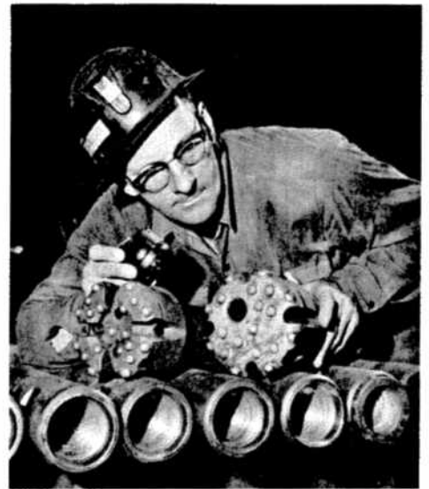
Mine foreman Al Maskell examines the tungsten carbide buttons on one of the bits used in down-the-hole drilling. The bits are pictured here on top of extra sections of drill rod or tube.
