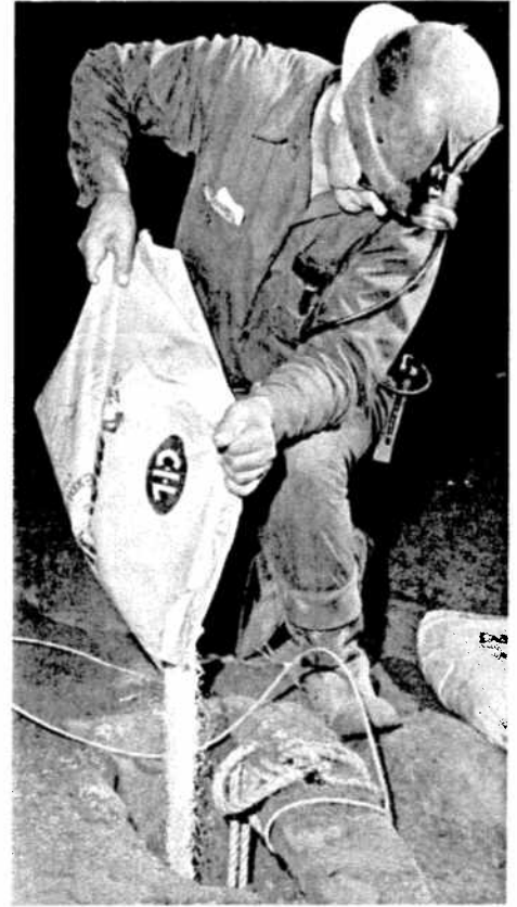
The blasting agent "Amex" is poured into the hole. When the required amount of "Amex" has been loaded a blasting cap is spliced to the prima-cord, then a final packing of sand tamps it all in place.
