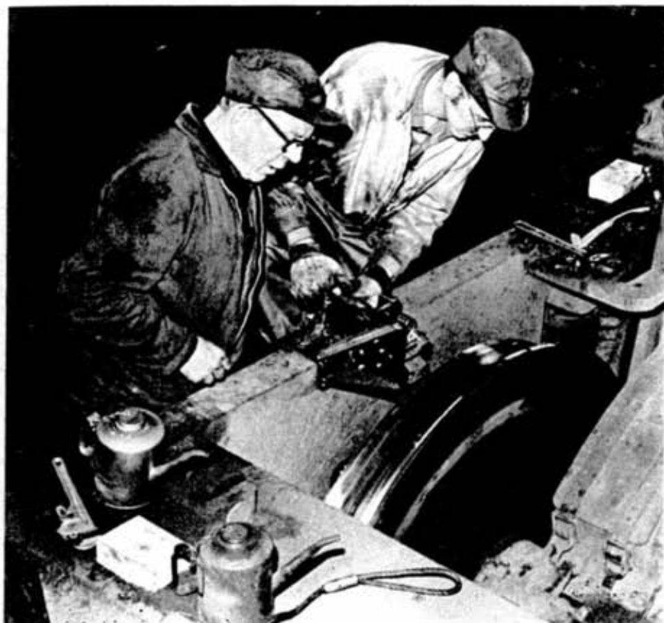
Del Briscoe and machinist Henry Lewandoski prepare to adjust the cutting tool to trim back the roll-over from the rim of the tire.
