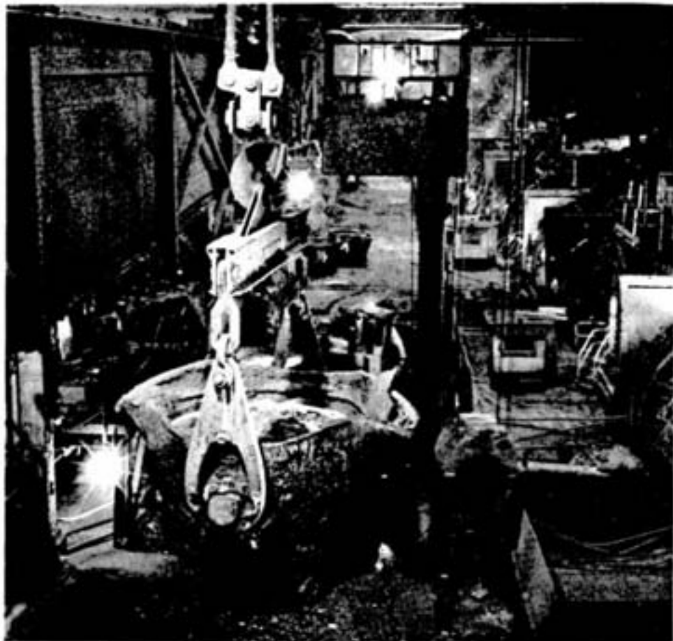
Len sounds his warning siren each time his crane prepares to hoist a ladle. Behind each of the spark shields is a converter which takes reverb furnace matte and produces a high purity nickel-copper matte.
