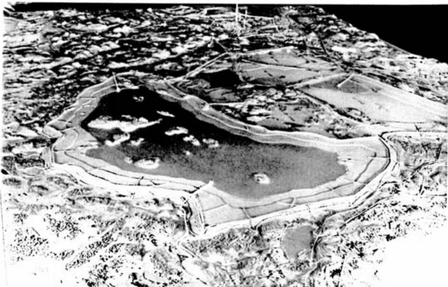
"R Area" in the year 2000: This view from Creighton, shows the landscaped terraced dams, as well as today's existing facilities in the right background. If the company's proposal is accepted, "R Area" will be able to accept all the tailings produced until the turn of the century.
