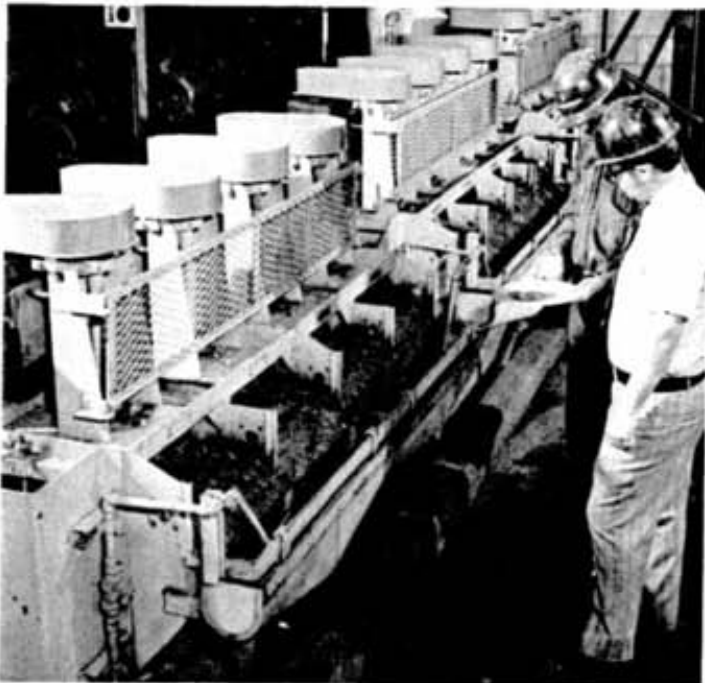
Brian Lyons and John Jazymantas are "panning" to obtain a quick sample of the mineral composition of the froth. Their "panning" is identical to that used by old-time prospectors for gold.
