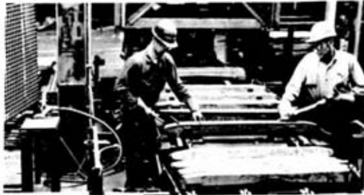
At one of the inspection stations, Harvey Bailey and Bill Flynn remove minor surface imperfections and check sizes of horizontal wire bars.
