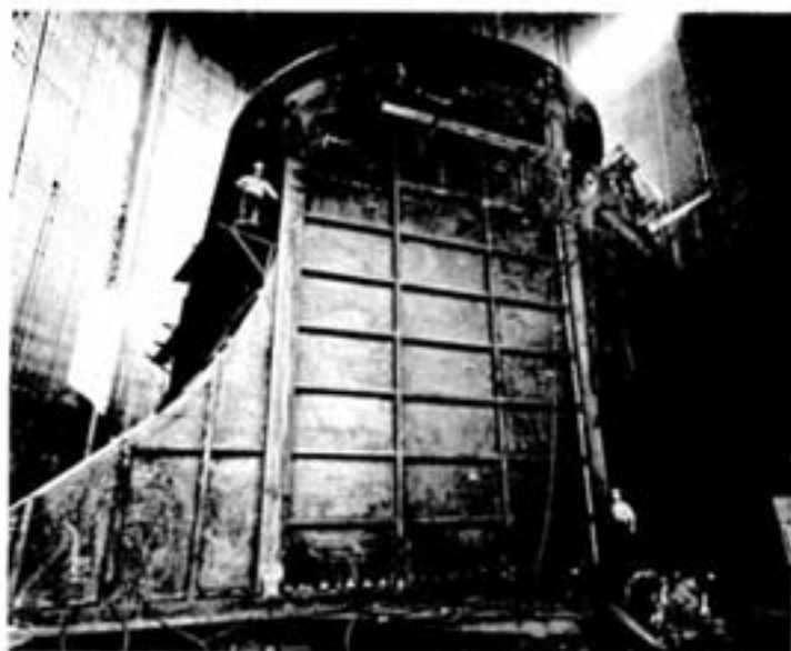
Inco's 1,250-foot superstack is now almost 90 per cent complete and will be on-stream the end of August. The stack's largest lift ever was recently hoisted to the bottom of the liner. It's this 110-ton transition piece which bridges the breeching and liner. Work remaining on the stack includes installation of electronics in the electrostatic precipitators, and the completion of the breeching which attaches to the stack flues.
