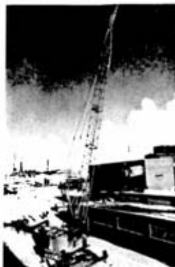
A 55-ton rated mobile crane, the largest crane on wheels in northern Ontario, was used to hoist one of the three-ton heating units onto the tankhouse roof. The crane has a 120-foot main boom, and a 30-foot extension, or fly jib, on which the heater is hanging.
