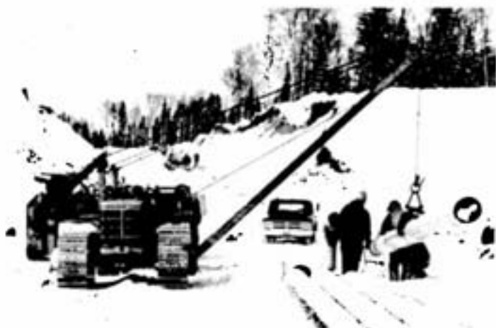
Nearly all of the tailings lines will be buried underground, as part of Inco's efforts to remain as unobtrusive as possible in the Lake Shebandowan area. Where burying is impossible due to the contours of the land, attractive trestles will be used to bridge the gap between tunnels.
