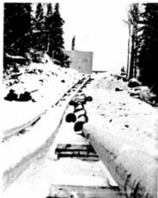
Over 10,000 feet of tailings lines will extend from the mill to the special 280-acre tailings pond Inco created to hold mill wastes. All mine water is treated on the 2300 level underground, and is then pumped 1½-miles for release into nearby Gold Creek, through the second pipe. The third pipeline returns the tailings effluent to the mill.
