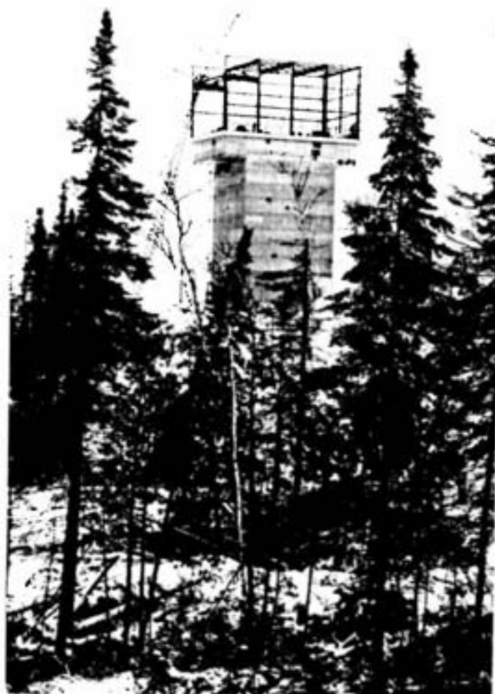
Framed by trees, Shebandowan's No. 2 shaft headframe is clean and uncluttered. In the final stages of construction, the concrete headframe will be 176 feet high and will house two 15-ton friction hoists in its penthouse. No. 2 shaft is 2,395 feet deep and the mine has a design capacity of 2,900 tons-per-day when it starts production in November 1972.
