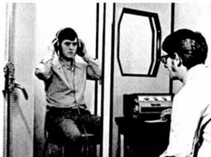
Assistant X-ray technician John Dandenault briefed employee prospect Jocelyn Corriveau, from Gaspé, Quebec, on what to expect and is about to conduct a hearing test. The two electronic "audio boxes" were added during the renovations. John dials a high-pitched whine into either headphone to determine the prospect's hearing range.
