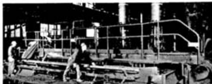
A general view of the top of the No. 1 electric arc furnace in the Orford building, this picture clearly shows the cable and pulley mechanisms that support the furnace's three graphite electrodes. At right, the open uptake allows free air to dilute and cool exhaust gases from 2,000 to a handleable 300 degrees F. Tending one of the furnace's two oscillating pan feeders are Claude Ranger and Joe Chaj.
