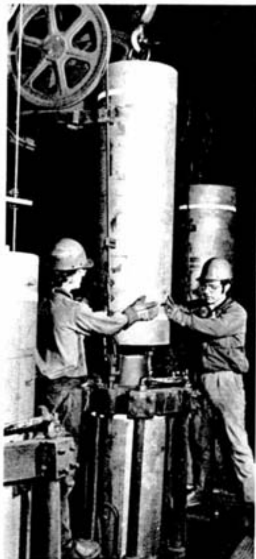
These are the furnace's three electrodes. Made of graphite, they extend down through the roof of the furnace to within one inch of the molten bath. The powerful electrical current they carry arcs between electrode tips and bath generating melting temperatures of close to 4,000 degrees F. As the anodes burn away they are lowered into the furnace and additional sections are added. Screwing a 6-foot long, 1,200-pound section into place are Dan Lewis and Joao DaSilva.
