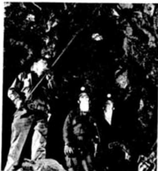
Making personal contact with drillers Tom Lacroix and Spencer Eloffson in the 27 crosscut, Bill demonstrates the established safe method of sounding for loose.
