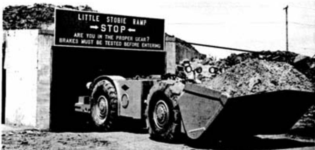
Entering the mine portal and heading down the ramp, this husky load-haul-dump machine is carrying a 7-ton load of crushed rock that will be used for road bed. Driven at an incline of 20%, the ramp is 16 feet wide and 12 feet high. Now down to the 600 level, the winding road is 3,250 feet long.
