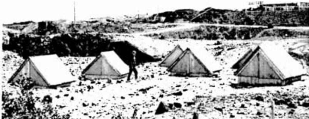
Each of these huts houses the upper ends of six stainless steel wires. The lower ends of the wires are anchored in the hangingwall close to the Little Stobie orebody on the 100-, 150-, and 200-foot levels. A ground control system, they monitor rock movement during the preliminary stages of sub-level caving. Using extensometers to measure changing strains in the wires, engineers are able to plan precisely controlled caving of the hangingwall rock.
