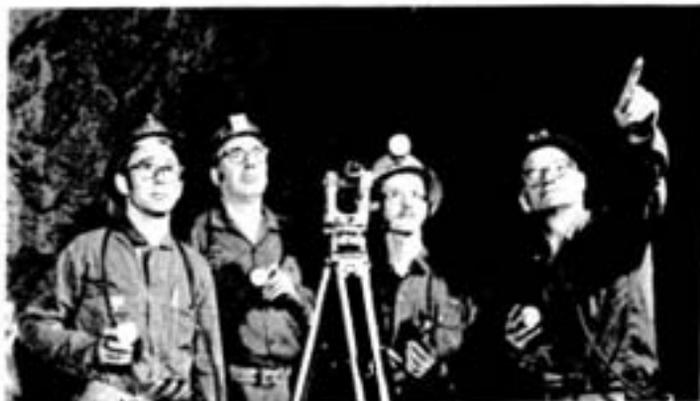
On the 50 level while on an inspection tour, Mine Engineer Don McLeod and Little Stobie Mine Superintendent Sam Pataran are seen with Survey Assistant Gerry MacIsaac and Layout Engineer Charlie Pitts. The survey instrument was being used to install lines for ring drilling.
