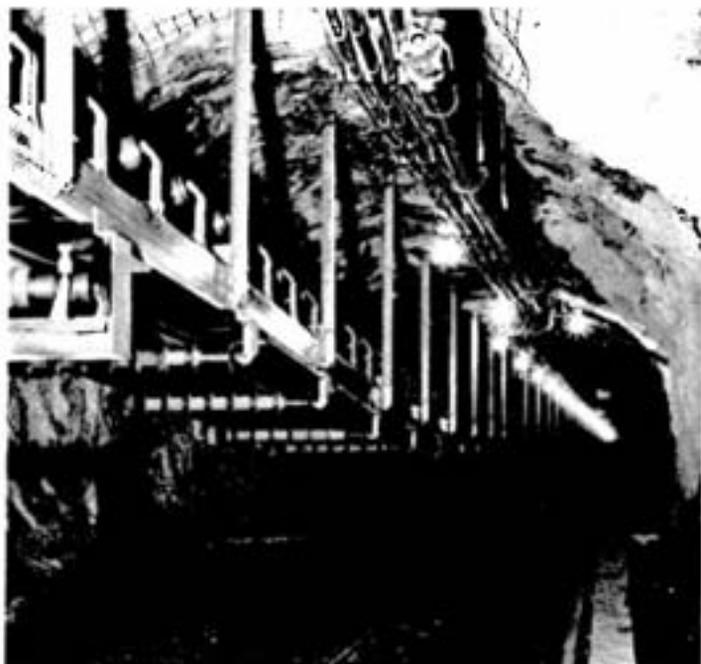
Nearly a mile long, this 42-inch roof-suspended conveyor is located on the 2400 level and carries ore from Little Stobie Mine to Frood-Stobie No. 9 shaft. With a belt speed of 481 feet per minute, it can deliver 1,000 tons of muck per hour. It is powered by a 250-h.p. motor. The endless belt has a total length of 9,400 feet, weighs 1,034 tons, and carried a price tag of close to \$200,000.
