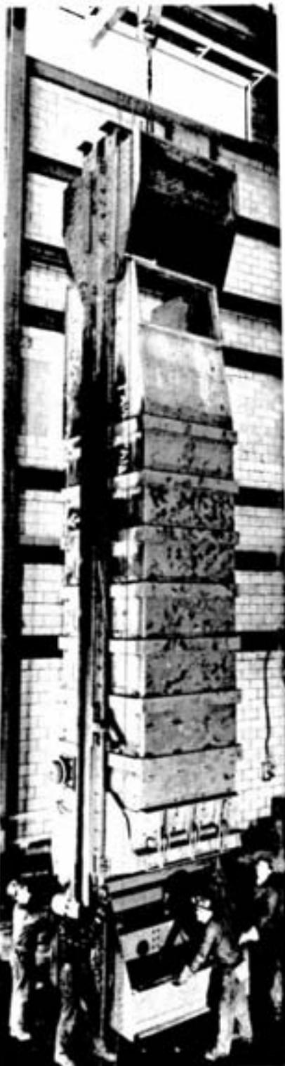
In the collarhouse at Frood-Stobie No. 9 shaft, this is one of the 20-ton bottom dump skips, largest in the Ontario Division, in which Little Stobie Mine ore is hoisted to the Frood-Stobie Mill storage bins. Operated by a 4,200-h.p. 4-rope friction hoist, the skip travels at 3,000 feet per minute. Dwarfed beside the huge conveyance are Riggers Frank Kuznik, Moses Roy, Tony Pinard and Gerry Vincent.
