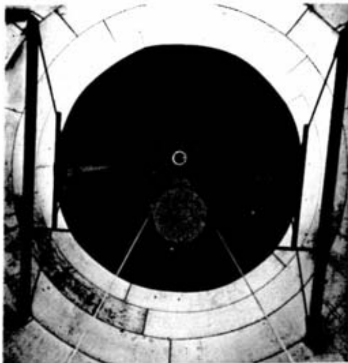
A WORM'S-EYE VIEW inside first section of steel liner, showing the man cage ascending and, almost a quarter of a mile up, daylight filtering around the liner installation platform at the top of the stack. Detachable steel framework on liner is for hoisting.
