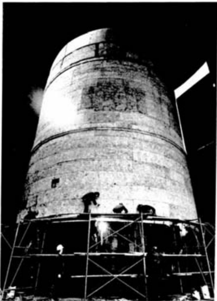
WELDING THE bottom ring and applying fibreglass insulation to first section of 2,000-ton liner before hoisting it to the top of the super-stack.
