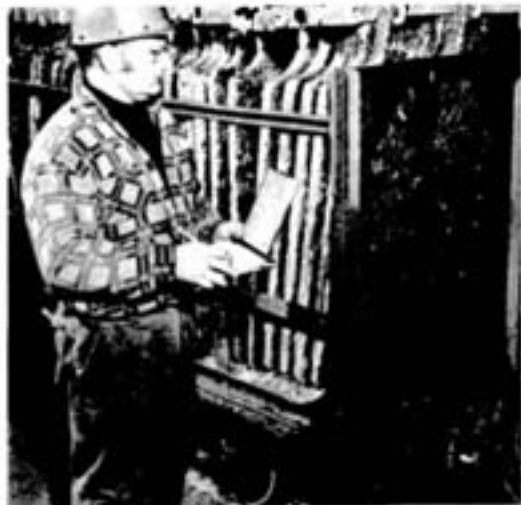
Suspension bar bolted to the lugs, a still-hot anode is hoisted from the casting wheel by floorman Joe Zdelar. On the right, weigher John Mikolasek checks out a car of anodes on its way to the final refining process in the electrolytic department.
