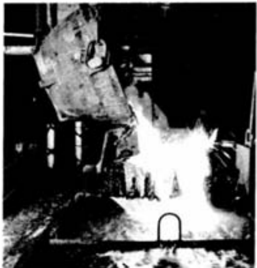
Molten furnace slag is poured on high-pressure jets of water which granulates it into shot, convenient to handle in further metal recovery treatment. On the right, anode department superintendent Jan Van Dillen (with pencil) confers with assistant to the superintendent Les Way and assistant superintendent Lloyd Schooley on a refractory problem.
