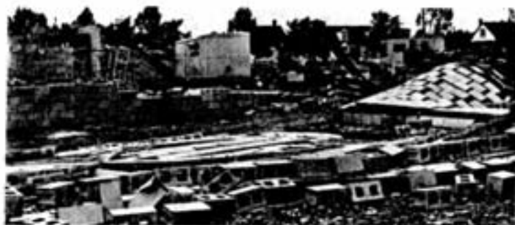
Walls were flattened in heavy damage to $1¼-million extension under construction at Lively High School.
