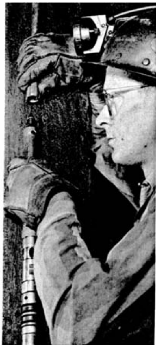
WITH HIS RIGHT HAND, drill helper Bob Legault has depressed the lifting dogs of the overshot to disengage the spearhead of the core tube assembly. The dark rings in the assembly are the rubber shut-off valves which expand under pressure when the core tube is filled.
