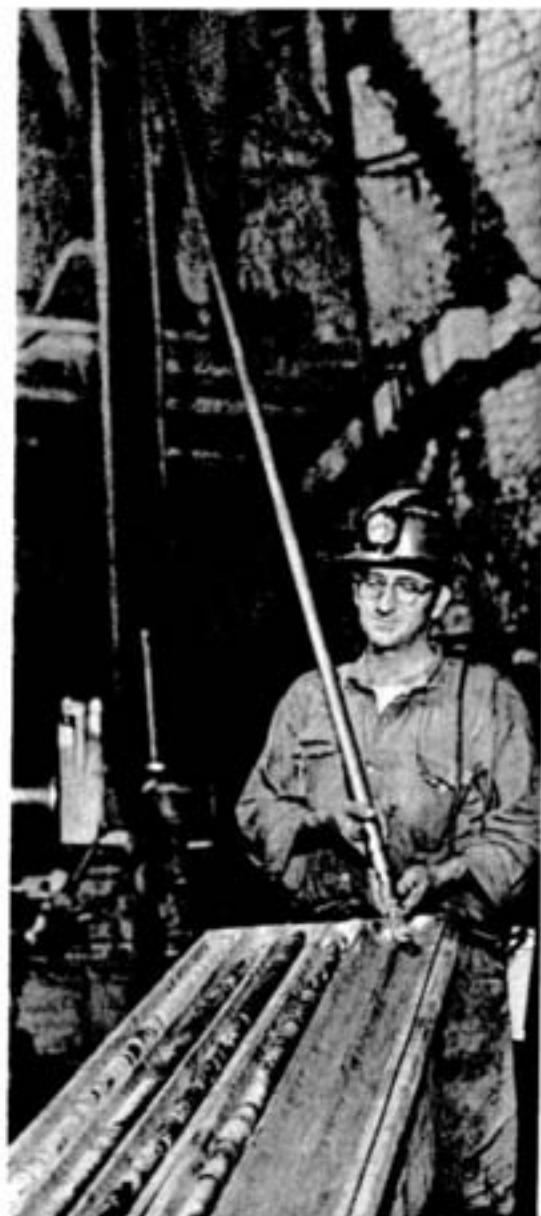
ERNIE MYRE is emptying the \frac{3}{4} -inch drill core from a 15-foot tube into a core box which, identified as to the location and depth of the hole, will be sent to surface for examination by exploration geologists.
