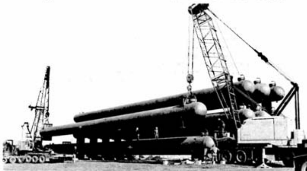
An indication of the size and complexity of installations for the IPC (Inco pressure carbonyl) section of the new nickel refinery now under construction at Copper Cliff, to cost in excess of $100 million, are these huge pressure storage tanks for process gas. Manufactured in Toronto, the 120-foot tanks each required three railway flat cars for shipment, and were delivered from the railway to the plant site on specialized lowboy equipment. Fifteen tanks of this size are involved in the installation.
