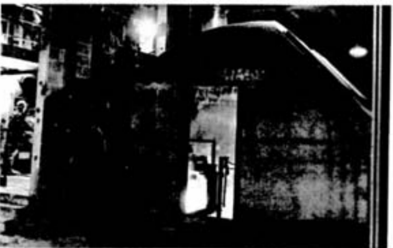
Fibre-glass hood over the slag granulator pit is known as "the pumpkin".
