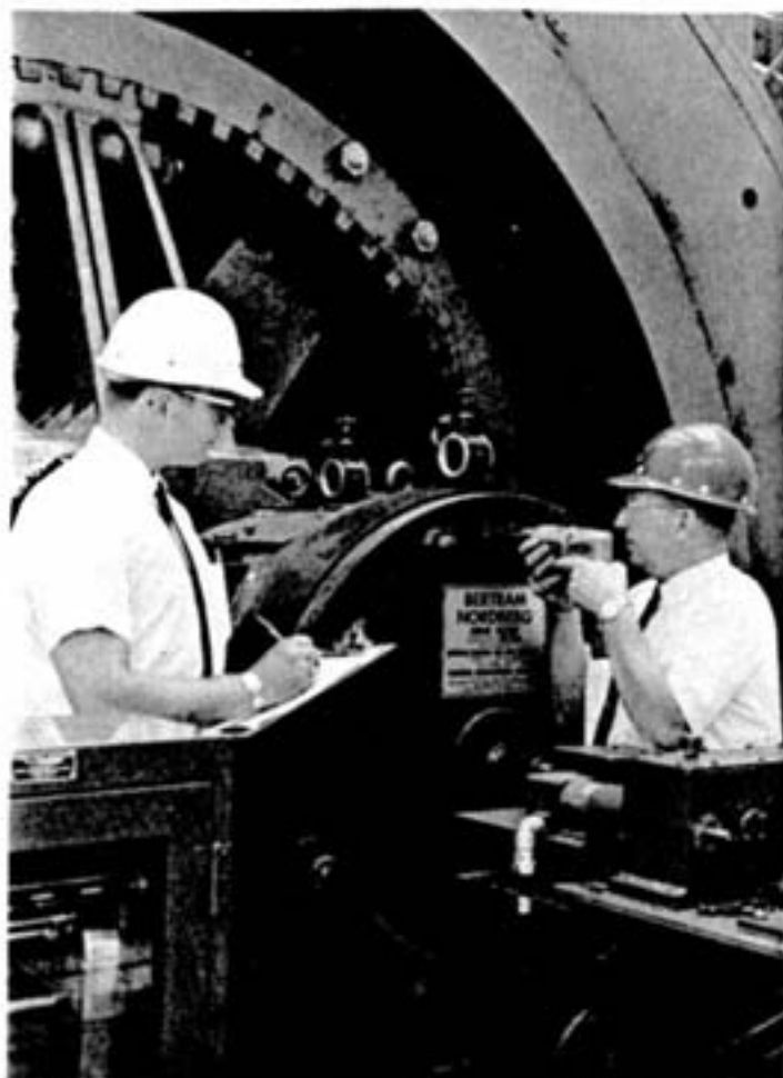
All items of permanent equipment, totalling many thousands and ranging all the way from the huge electric shovels at the open pit down to the lowliest sump pump, are identified by the property and insurance section with a numbered metal plate. Here John Flynn attaches a plate to the new hoist at Copper Cliff North mine, one of the largest hoists at Inco. Recording the identification is Ray Chateaufort.
