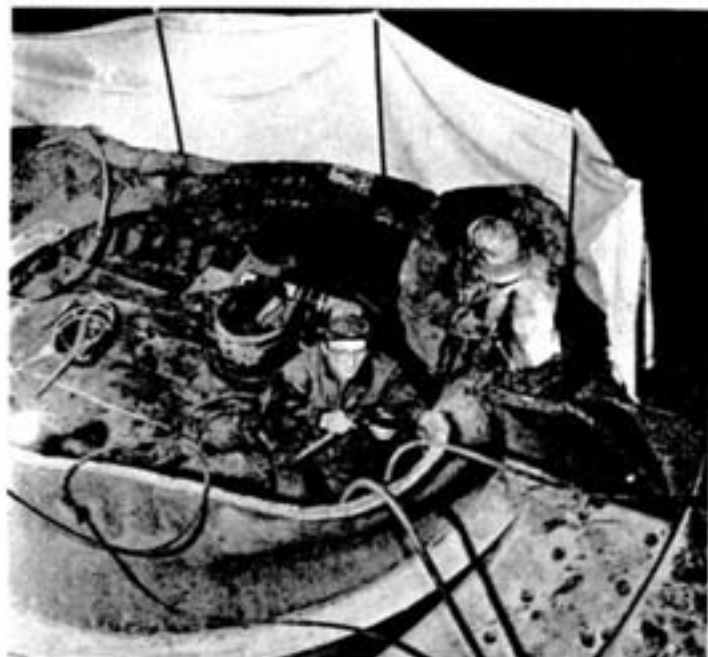
Among the heavier equipment that the department maintains are the big smelter converters, 13 feet 6 inches in diameter by 35 feet long. While down for re-bricking this converter is having its collar cleaned up and rebuilt by welders Orest Kalinski and Micky Vicente.
