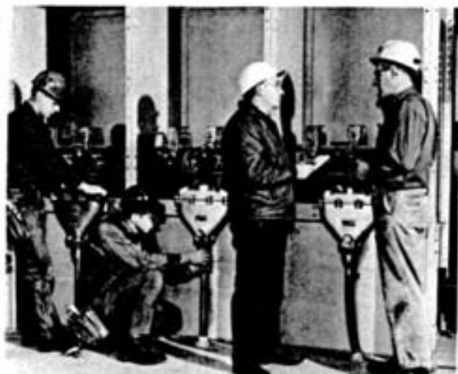
Also responsible for the installation and maintenance of the electrical power distribution system, members of the department are seen here installing the 13,800-volt pot heads in the recent extension of the smelter compressor building. Finishing the job are electrician helper Milton Rodar, electrical apprentice Paul Puga, maintenance supervisor Harry Lamontagne, and lineman John Hacquoil.
