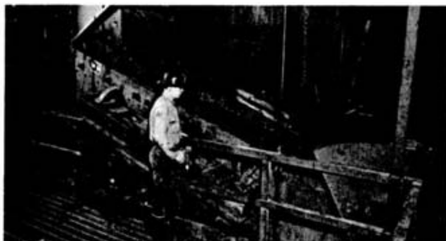
Incoming sand feeds from the receiving bin to a vibrating screen. Screened sand drops into a 3,000-ton storage bin immediately below. Barry Connors is seen making a routine inspection of the screening operation.
