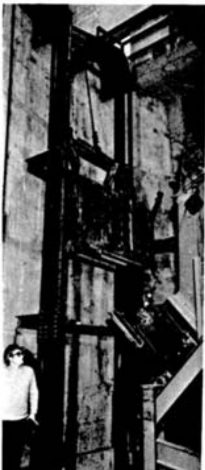
Oversize material is rejected by the vibrating screen to a small automatic skip which returns it to surface for road and yard surfacing. On left is mining engineer Frank Russell.
