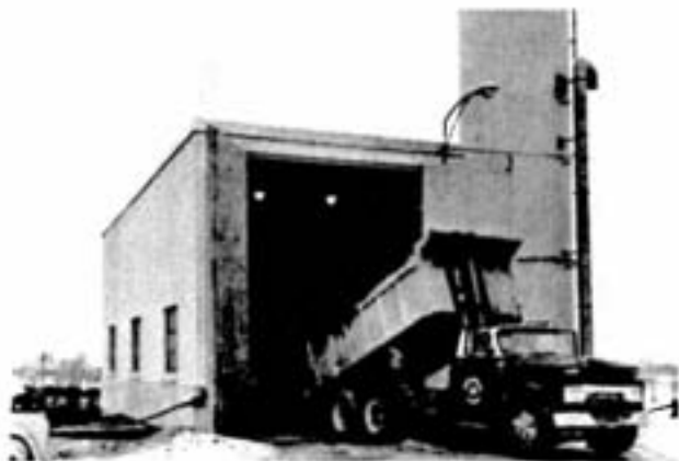
Sand from the pit half a mile distant is dumped into a receiving bin at the top of Garson's new sand plant. At rear is the 250-ton silo in which dry bulk cement is stored.
