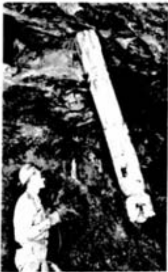
Diamond drill boss Larry Poulin inspects the break-through of the 11-inch pilot hole, less than 15 inches off target.
