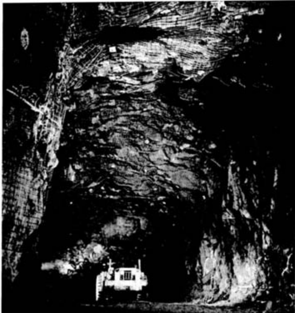
A powerful low-slung ScoopTram with a 5-ton load of ore in its bucket moves smartly from muck pile to ore pass in a cut-and-fill stope just above 800 level at the Frood. The low camera angle accentuates the height of the big stope, which is 20 feet. Clearly shown are the extensive roof bolting and wire screening, standard protection in this mining operation. The cemented sand fill floor provides ideal travel for the trackless mining juggernaut, which puts on a demonstration of ore removal that would make the old slusher sigh with envy. You can't see him from here but Joe Jackson is at the controls.
