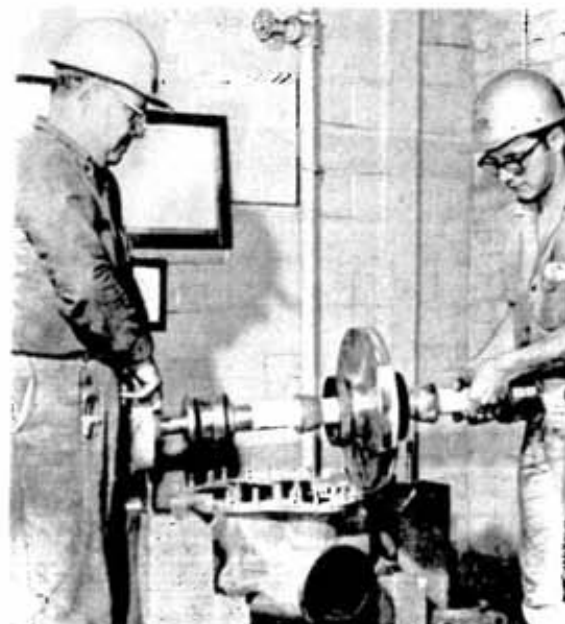
Electrician apprentice (3rd year) Wayne Totten assembles a cooling fan under the watchful eyes of Archie McIntyre, maintenance electrician 2nd class, who has a thorough knowledge of all the small motors and electric tools used in the plant.
