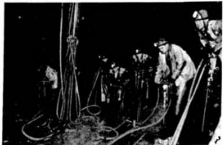
PART OF A NINE-MAN CREW, using hand-held pluggers, are shown drilling off a 10-foot bench at the bottom of the shaft. The drills, with hoses attached, are stored on the stage when not in use, and are lowered to the shaft bottom by a tugger hoist. Shaft sinking operations at Creighton 9 are on a seven-day round-the-clock basis.
