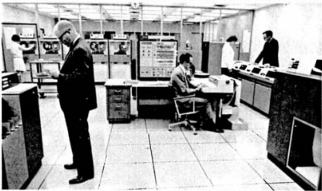
each. In right foreground is the high speed printer from which come all reports requested from the machine at the rate of 20 pages a minute. The printer also prints employees' pay cheques at a speed of two per second.
