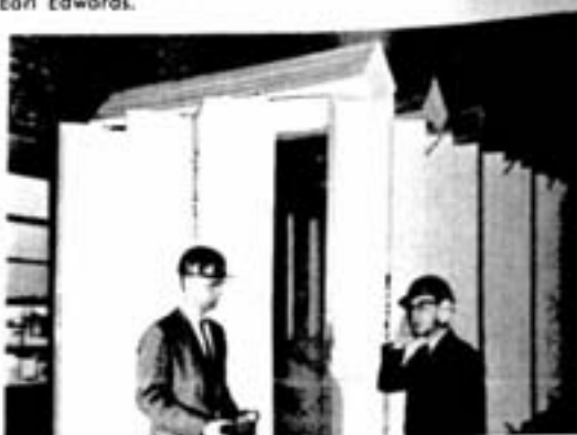
Using an octave band noise analyser Lloyd King, general foreman, and Gerry Martin, noise abatement engineer, are measuring the total sound pressure created by rivetting in the Copper Cliff plate shop. At left is smelter safety engineer Harold Waller; rivetting are plateworker Amio Tonelli and helpers Norbert Lalancette, Earl Edwards.
