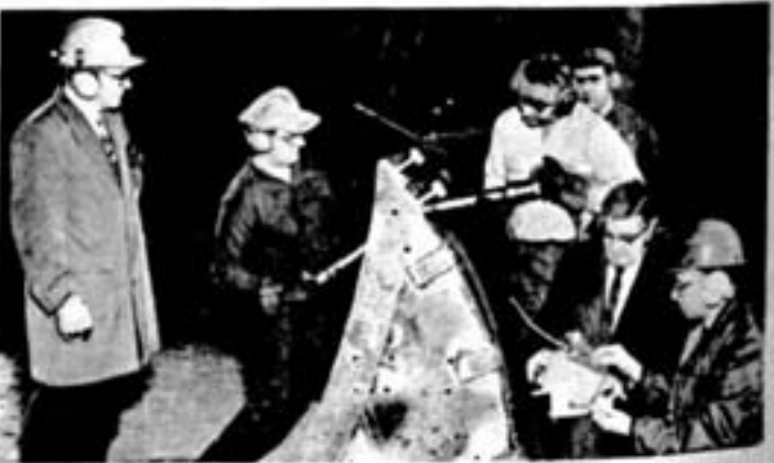
Using an octave band noise analyser Lloyd King, general foreman, and Gerry Martin, noise abatement engineer, are measuring the total sound pressure created by rivetting in the Copper Cliff plate shop. At left is smelter safety engineer Harold Waller; rivetting are plateworker Amio Tonelli and helpers Norbert Lalancette, Earl Edwards.
