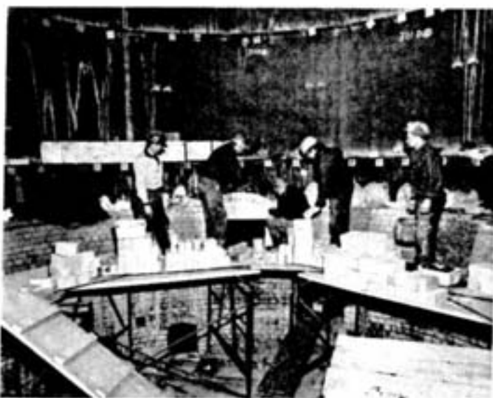
TAKEN INSIDE THE NEW ROASTER, this picture shows initial stages of installing insulating material and firebrick to protect the huge steel shell in which concentrate filter cake is partially oxidized to a calcine at temperatures about 1200 degrees. Inco mason Frank Gramolini is inspecting progress.
