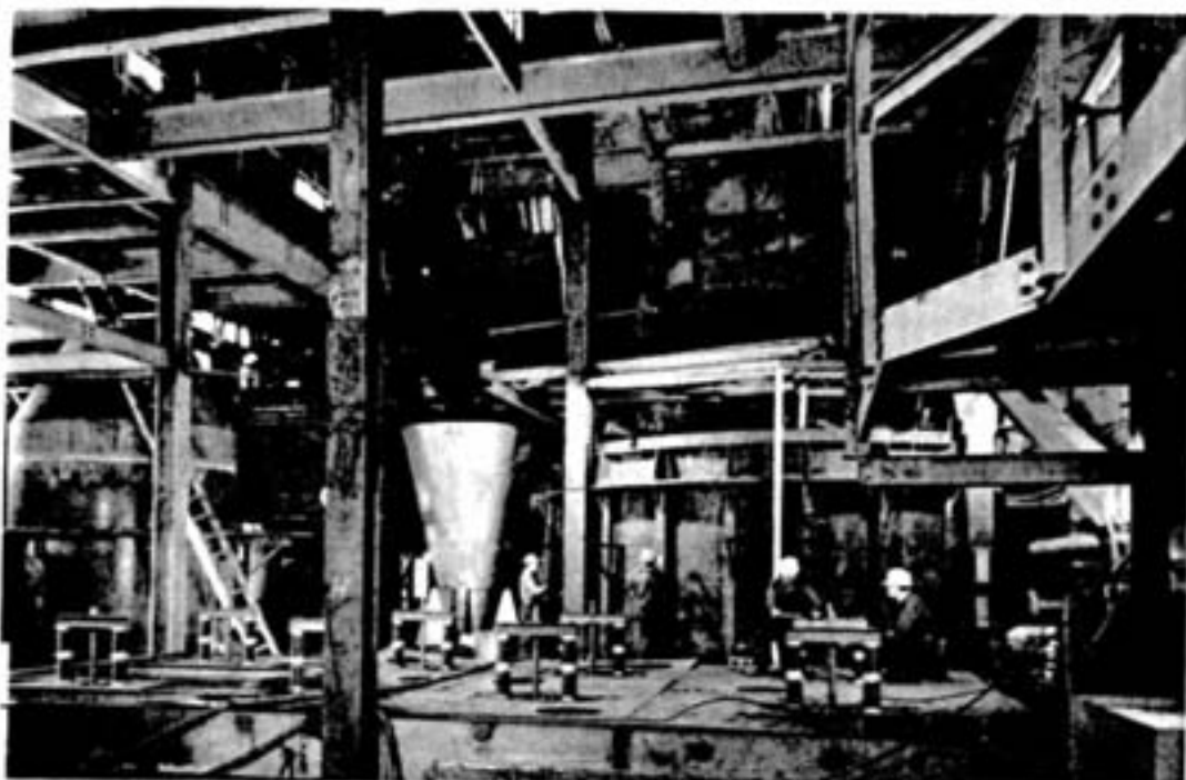
PART OF THE SMELTER REVERBERATORY DEPARTMENT'S first new fluid bed roaster is shown under construction in this photograph. The cone-shaped object beside it is a section of one of two dust collecting cyclones which clean the roaster gases. On the left is the heat exchanger in which the roaster gases are used to pre-heat the incoming blast air required for the operation of the roaster. The area on which the men are working is the top of the roaster's electrical precipitator.
