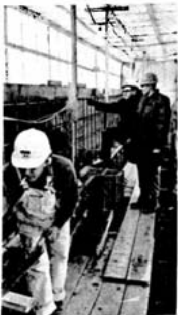
Polyethylene hoarding, boon to cold weather construction, provides workmen with green house conditions while the temperature is 40 below outside. Here assistant chief engineer Ernest Kolmanovitch discusses steel framing of the exterior walls for the warehouse extension with Ron Coleman, Molcom Construction Company's construction superintendent.
