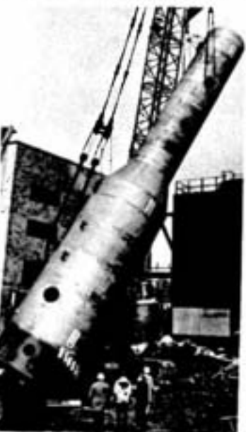
This was the scene in April of last year as the 75-ton main distillation column of the oxygen plant's new unit was being positioned on its concrete pad. Clad with nickel stainless steel it is 70 feet high.
