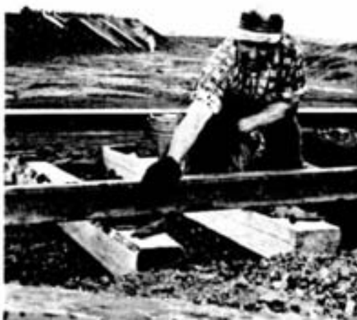
Valentino Basso aligns tie plates on new ties. In background slag is being poured on No. 3 dump.
