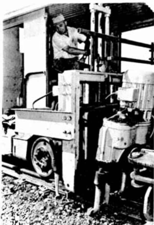
Electromatic tamper exerts a 7000-pound downward thrust on its 16 penetrating tools to compact the ballast around relocated track. Operator shown is Angelo Demarchi.
