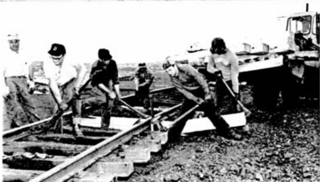
The track gang replaces damaged ties and trims the crushed slag ballast after the track is shifted.
