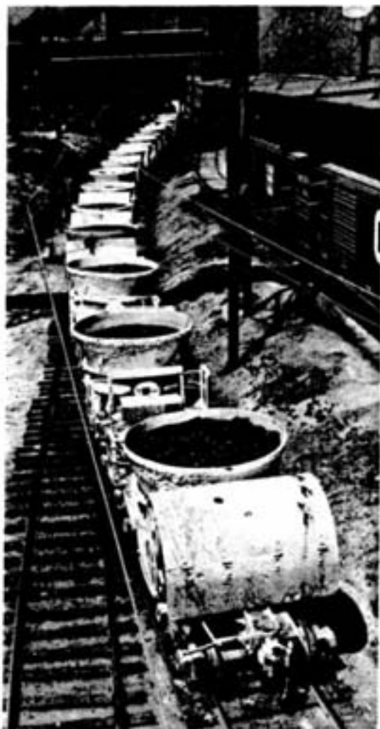
A 17-car slag train moves out of the smelter on its way to the dump. Each pot holds about 16 tons.
