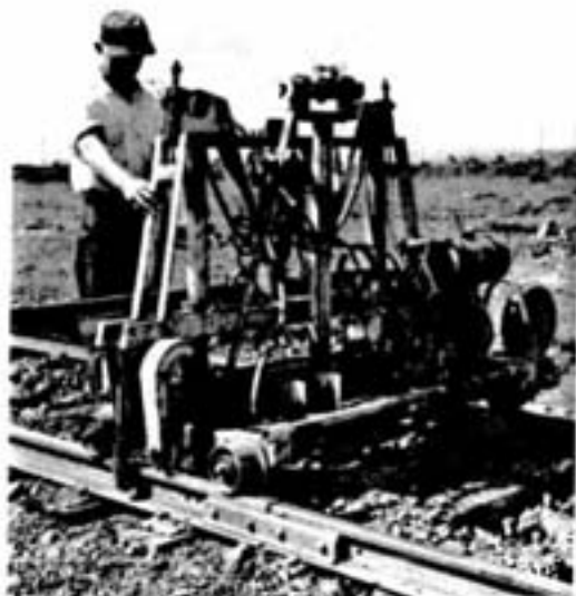
This power jack is used to correct the cross level of relocated track.
