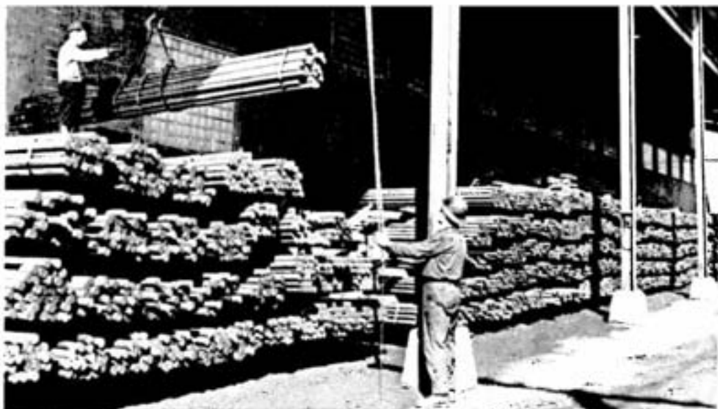
INDICATIVE OF the tremendous quantities of grinding media required to feed the maws of the ever-hungry mills at Copper Cliff is this storage shed which houses 1,200 tons of high-carbon steel rods, about three months' supply. Picture shows a bundle of 2½-inch diameter rods starting on their way to replenish a mill; receiving the appropriate hand signal from Aulis Vepsa, Leo Blais is operating the 5-ton hoist to lift the bundle.
