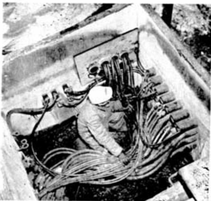
MORE OF THE "NEW LOOK" in the smelter; one of these control stations is located beside each of the five oxygen-using reverbs. Lionel Paradis is adjusting the coal-firing rate for number 6 furnace. Natural gas, oxygen and combustion air are also controlled from the panel.
