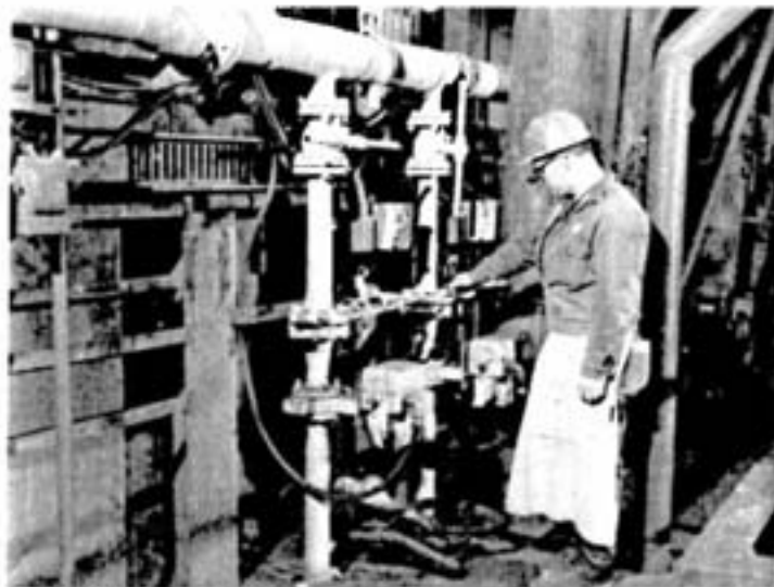
GENE AUGER, tapper helper at number 6 reverb, inspects the oxygen piping on C floor above his furnace. Controls for each oxygen lance include a manually-operated ball valve and an orifice meter as well as the butterfly flow-control valve operated from the furnace control panel.
