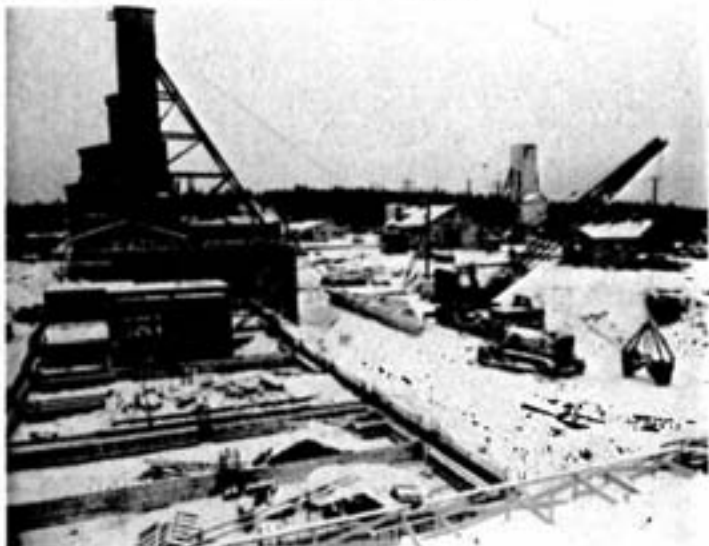
The temporary headframe and footings for the surface plant at Birchtree No. 1 are shown above. To the right is No. 2 shaft, which has been sunk to 1373 feet and is now being used for level development. It will become the air intake raise for the mine at the completion of development.
