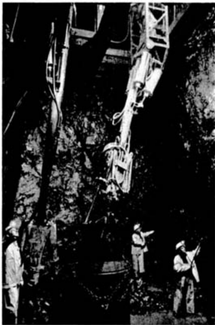
Two Cryderman mucking machines are being used in sinking No. 1 shaft at Inco's new Birchtree mine, three miles west of Thompson. The operator of one of the clams can be seen at top right in the picture. Two shaft miners are scaling down loose, and a third is signalling to have the bucket of muck hoisted. This 5-compartment shaft will measure 19 ft. 8½ in. by 14 ft. 5½ in. outside timber, and will be 2800 ft. deep.
