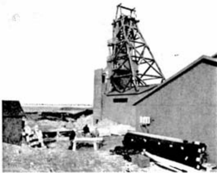
This is part of the surface plant at the new MacLennan mine, about 10 miles northeast of Garson, where the 3-compartment shaft is down about 800 of the projected 1050 feet. Slope production is scheduled for next June at the rate of 800 tons per day. Open pit mining at MacLennan, commenced last May, will be completed next summer; the ore is being shipped to the Copper Cliff mill.
