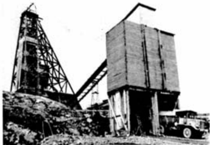
A view of the headframe and ore bins at the Totten mine No. 1 shaft, half a mile southwest of Warthinton, where sinking and development work are completed and the mine will commence production early in 1966. Totten No. 2 shaft, 1800 feet northeast, has been collared and the sinking plant is now being erected. It will be 2000 feet deep.
