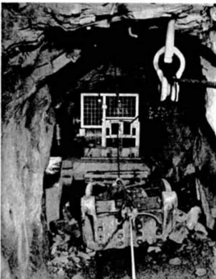
Here's a view of a working place at Frood-Stobie, one of 60 such active slusher drifts in the Stobie section of the mine. The operator shown, Albert Leroux, stands at the controls of a 125-hp slusher hoist with which he skilfully manipulates a 72-inch scraper to pull broken ore through a draw-hole into mine cars standing on a track below. Ore enters the drift through boxholes spaced at 33-foot intervals along each side. The length of the drift varies according to the width of the orebody, and may be up to 300 feet.
