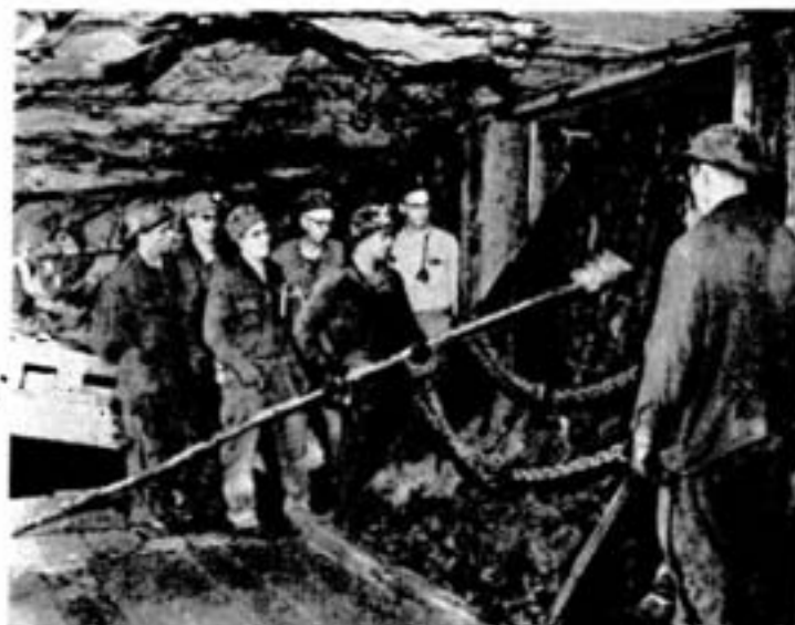
9. Another strong feature of the safety program are daily job demonstrations scheduled by the shift boss and carried out under his direction. Members of senior supervision also attend. In this demonstration the correct method of making up and placing a blast in a hung-up chute is being shown by pillar leader Henry Piche. Others in the group are, from the left, stope leader Andy Luyten, raise driller John Laverty, shift boss O'Malley, divisional foreman Sunquist, underground superintendent Milt Jawsey, and, on the right, stope leader Leo Barrette and raise driller Ed Carre.
