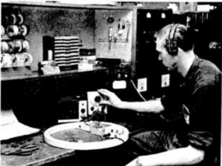
1. GROUND CREWS GO IN to make a follow-up investigation of an area where interesting geological indications have been reported by the air-borne geophysical survey. Technologist Gord Jinks is shown here building an electro-magnetic transmitter that may see action this summer in the barren lands. 2. Companion piece to a transmitter is the pickup coil used to
