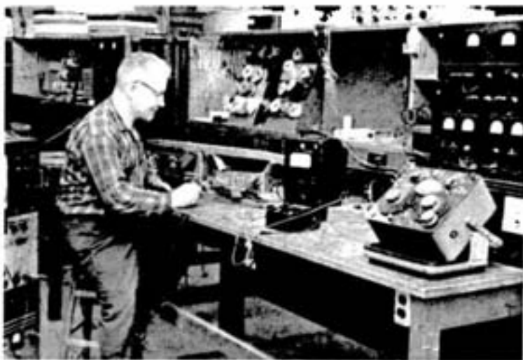
1. SURROUNDED BY A BATTERY of impressive-looking test equipment technician Nick Mandziuk is seen here at his bench in the geophysical research shop at the Froid hangar. He is constructing the delicate electronic apparatus for a "bomb" or "bird" that is towed beneath a plane in geophysical exploration to measure the electrical conductivity of the earth and report any irregularity which may be caused by mineralization. Inco was the first
