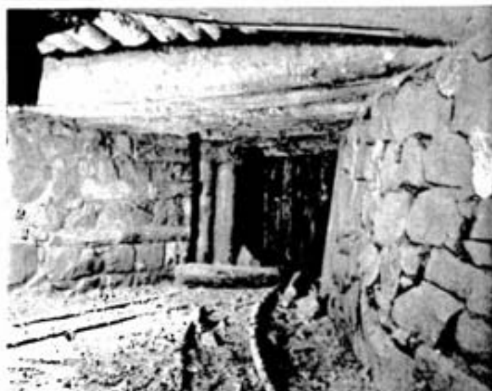
Native pine timbers were supported by dry wall in the old Crean Hill workings. Picture shows an intersection on 6 level, which was a main tramming level. After unwatering the dry wall and timbers were found to be as good as new.
