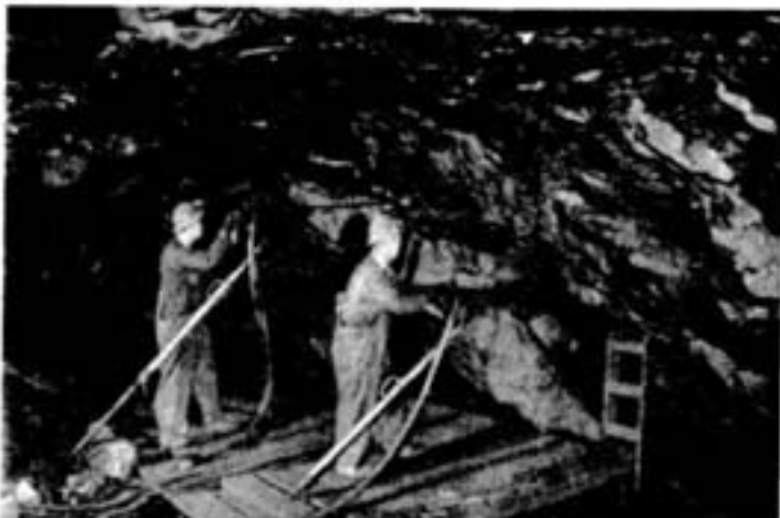
The 1000-level stopes are being mined by the shrinkage method with rock-bolting. Picture shows stope leader Ray Wheaton and driller Bob Elliott drilling off a portion of the breast in 10.9 shrinkage stope.
