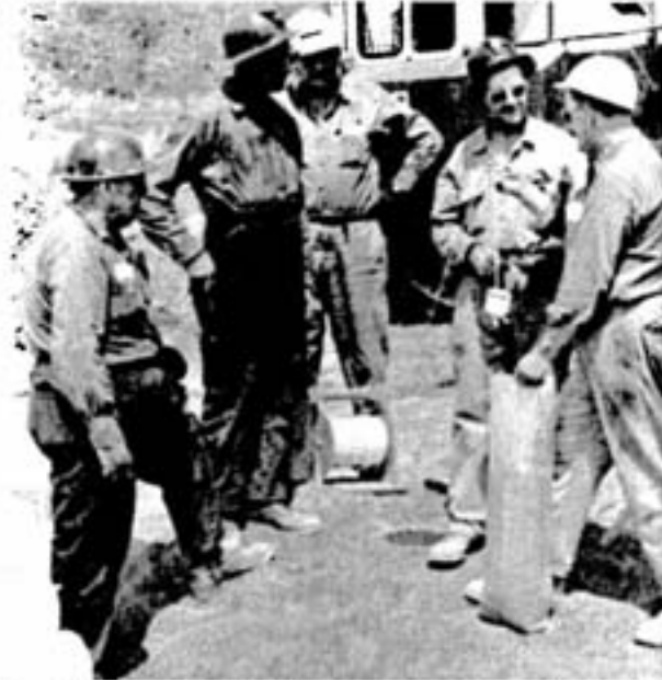
As at all Inco mines and plants, safety is an integral part of the operation. Seen here conducting a regular safety demon- stration is blaster boss Metro Rosko, who is showing bench blaster Frank Kangas the correct way to insert a primer in a 50-pound bag of explosive. Watching the demonstration are shift boss George Quigley, blaster Tony Muzzin, and pit foreman Bill Vaananen. During blasts all men remain in a blasting shelter.
