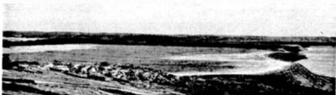
Another phase of the current tailings stabilization program is illustrated above; banks of tailings areas are being faced with crushed rock. The area shown is sown to grass but the banks were too steep for this treatment and were at the mercy of the wind until tied down with development rock from Copper Cliff North mine.
