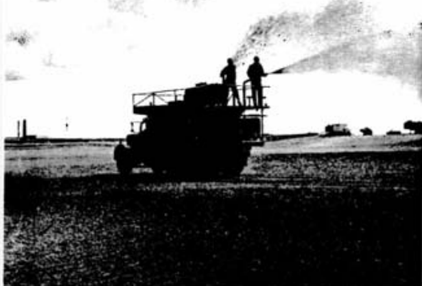
The mulch of low grade pulp paper, asphalt, fertilizer, grass seed and water is sprayed from a tank truck in the latest experiment in tailings stabilization at Copper Cliff. Picture on the right shows the low grade paper being fed
