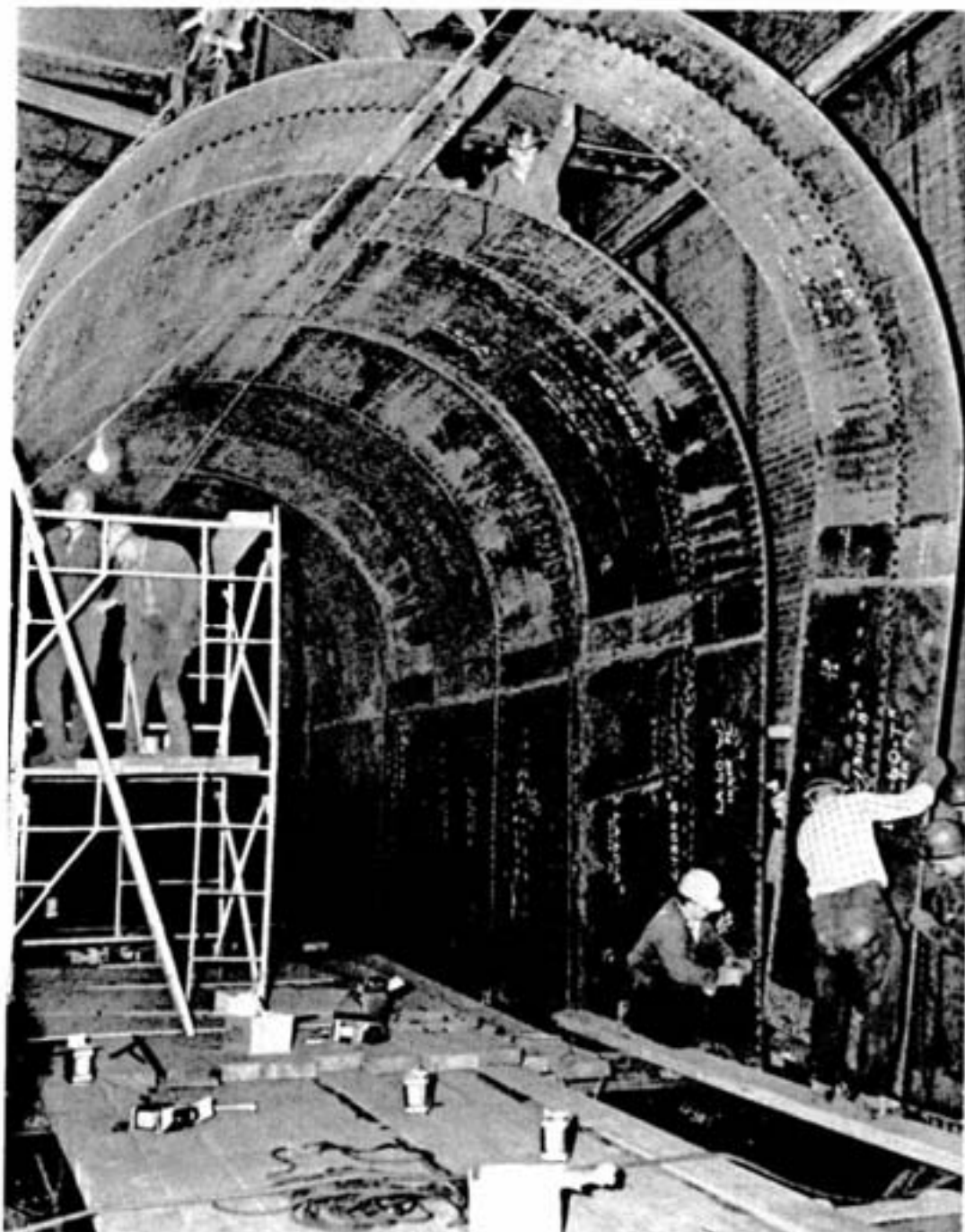
An 1800-pound plate of \frac{3}{8} -inch steel is seen being placed in position during installation of a new section in the converter flue at Copper Cliff smelter. A mobile crane and a trolley beam system were used to handle the 225 tons of plate involved in the job. Maintenance mechanics shown in this picture are (left) Les Delyea and George Clarke, (above) John Grant and Pete Zuliani, (right) Eddie Norquay, Harry Sawkiw, Conrad Page, Leo LaFreniere, and John Paquette. The work was carried out under the supervision of maintenance mechanics foreman Jack Beaudry and sub-foremen Johnny Tolonen, Alex Salo, and Don Young.
