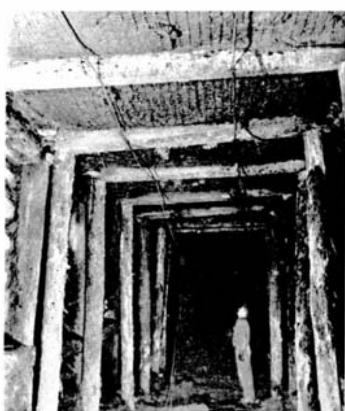
In this undercut-and-fill pillar on 1600 level at Frood mine the use of cemented sand fill has made it possible to replace laminated stringers and a solid log mat with a much simpler and less expensive screen-type mat supported on stringers. The miner is shift boss Jim Chisholm.
