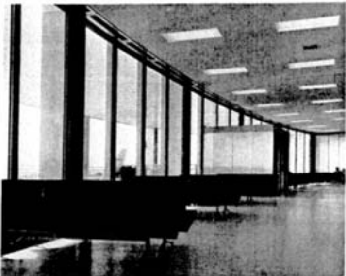
Nickel stainless steel curtain walls and siding on the entrances set off the 600-foot ring concourse of the aeroquay.
