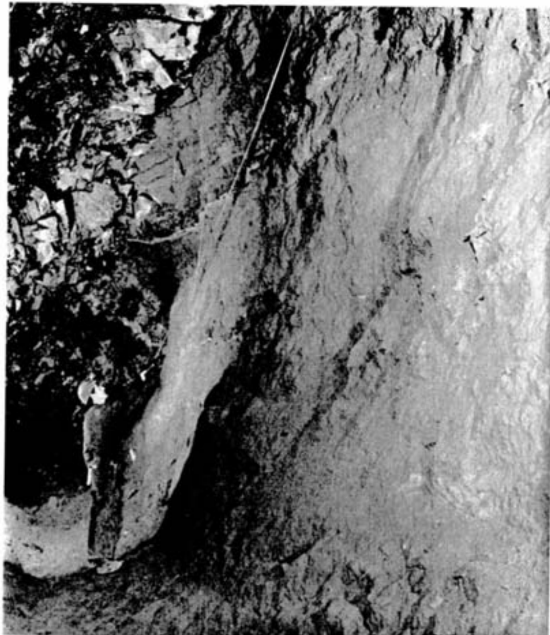
The trend to modification of existing mining methods made possible by the use of cemented sand fill is clearly exemplified in this photograph. Mining of a pillar is proceeding directly alongside a stope which was mined by the cut-and-fill method and filled with cemented sand. The height of the stabilized fill is approximately 20 feet, as indicated by the loading stick held by the miner. The additional strength of the fill allows the pillar to be mined by the more economical cut-and-fill method, as well as eliminating the necessity of a timber fence. The picture was made in 2972 stope on 1000 level at Frood mine during experimental studies in Inco's development of bulk filling with cemented sand. The miner is Roy Beaulieu.
