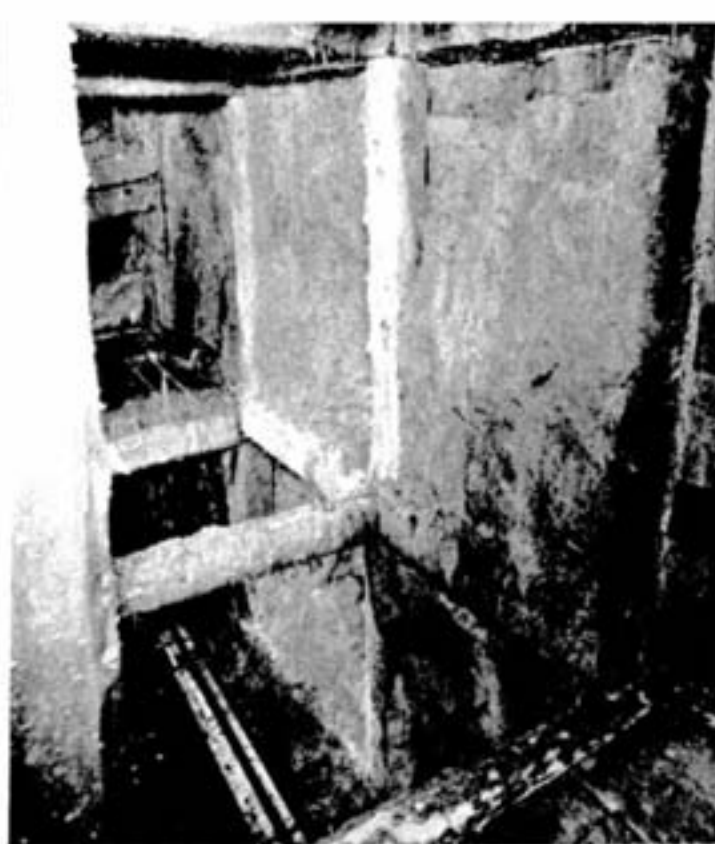
Here, on 3600 level at Frood, mining of a pillar is proceeding directly alongside a square-set stope section which has been filled with cemented sand. Prior to the development of the stabilized bulk fill, conventional timber fences would have been required to retain the sand fill.
