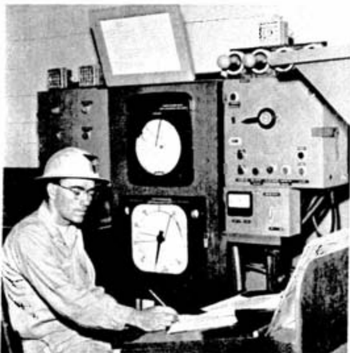
Here's the control panel in the Frood sand fill plant from which the operator regulates the ratio of cement to mill sands in the plant's mixing tank. A density gauge and a magnetic flow meter on the mixing tank outlet report automatically to the dials on the panel. The operator shown is Harry Shepherd.
