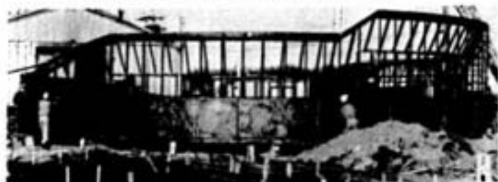
The cutting shoe was built upside down, then cut into sections and reassembled on caisson site. Note the varying elevations of the shoe's leading edge, which was designed to conform with the bedrock contours and varied as much as 8½ feet.
