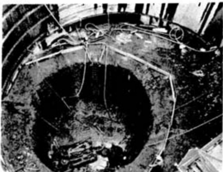
Bottom of the caisson after dewatering exposed the tremie concrete seal. The construction crew have commenced sinking the collar of the shaft. Close examination will show the contact between bedrock and the tremie seal.
