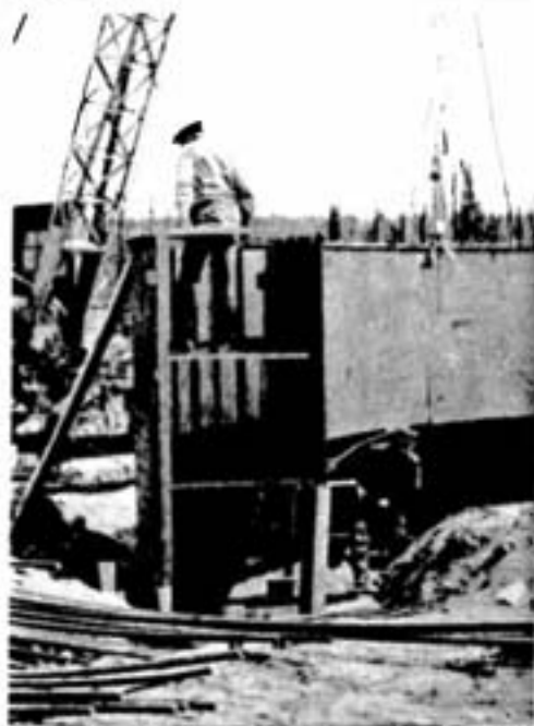
Picture shows the first section of the cutting shoe being adjusted on the gravel pad at the caisson site, the leading edge clearly visible. On the right a professional deep sea diver descends to clean the bottom and the interior haunch of the cutting edge as lowering of the caisson proceeds. The divers worked in muddy water with no visibility and at freezing temperatures.
