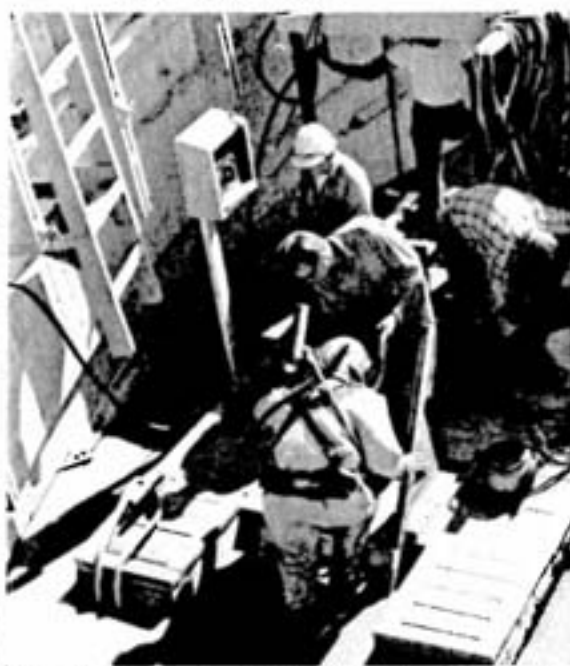
Picture shows the first section of the cutting shoe being adjusted on the gravel pad at the caisson site, the leading edge clearly visible. On the right a professional deep sea diver descends to clean the bottom and the interior haunch of the cutting edge as lowering of the caisson proceeds. The divers worked in muddy water with no visibility and at freezing temperatures.
