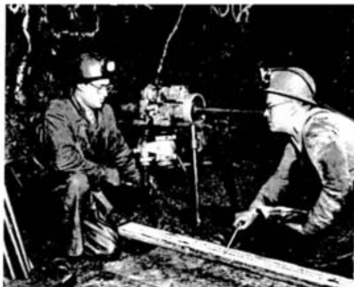
In 30 stope on 800 level Len Eckstrand checks drill core with driller Sacundio Rodriguez in a preliminary logging before the core is taken to surface for detailed logging and sampling. This visual check of the grade is to determine any change in the extent or attitude of the orebody, for control of mining operations.
