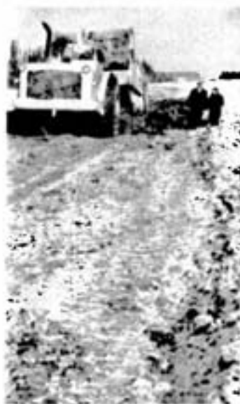
Four mammoth 36-yard Euclid earth movers like this are now at work on the Thompson-Wabowden link.
