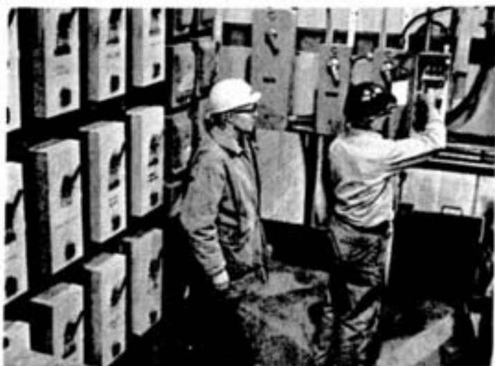
In no. 1 research station Don Armbrust is seen installing a motor starter. Watching is electrical foreman Eugene Bridge.
