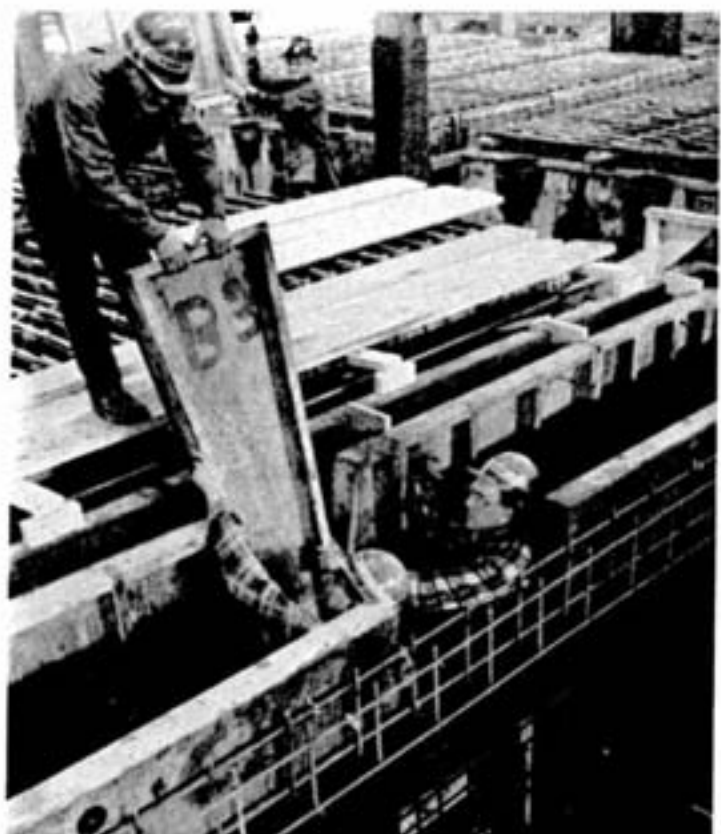
These men are installing forms to repair a concrete plating tank in the electrolytic department. Noel Marleau is handing down a form section to Walter Golding and Art Bonnar.
