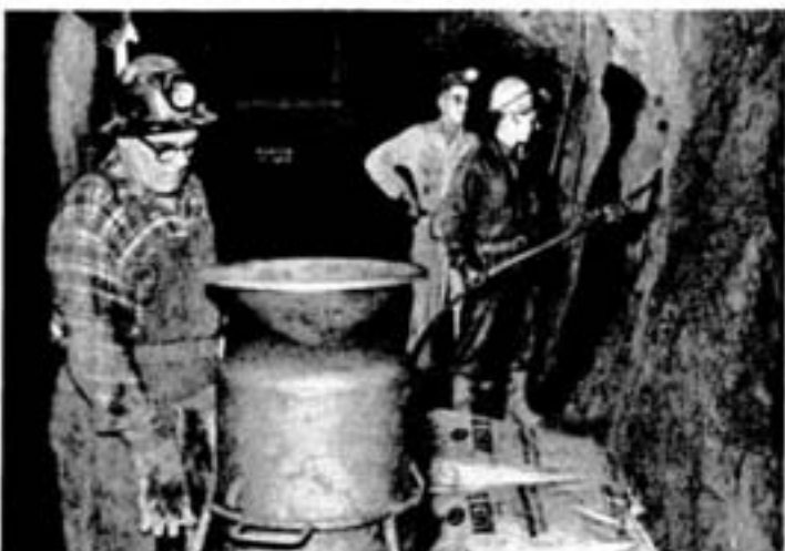
Loading longholes with blasting agent in a drill drift on 900 level: Ed Gauthier at the pneumatic loader, Bill Paquette on the hose, and shift boss Bill Stevenson in charge.
