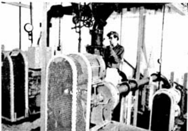
Each furnace has two sets of pumps for pumping the slurry of finely granulated slag from the granulator pit to the disposal area.
