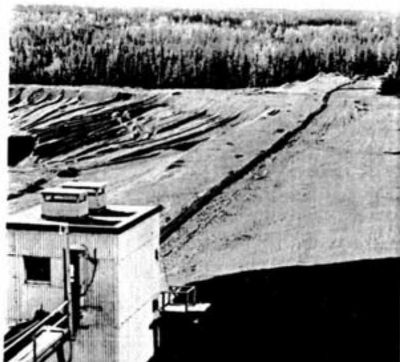
Each furnace has two sets of pumps for pumping the slurry of finely granulated slag from the granulator pit to the disposal area.
