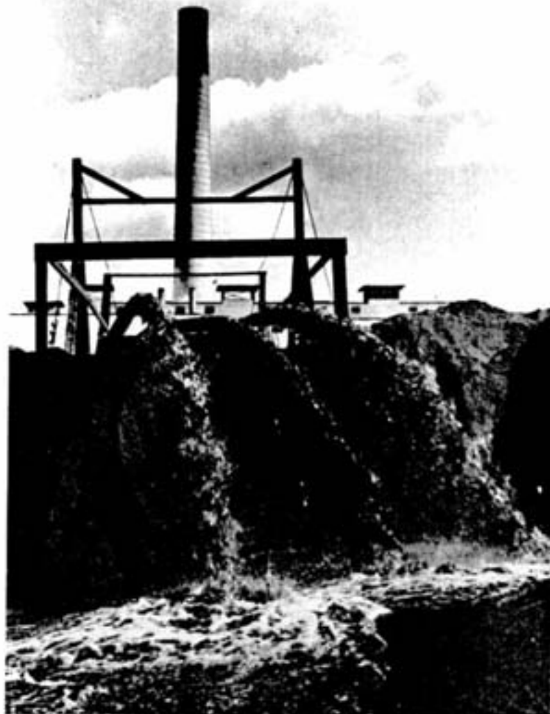
Three powerful streams of slag slurry gush from the rubber pipelines at the disposal area west of Thompson smelter at the rate of about 1000 gallons a minute.
