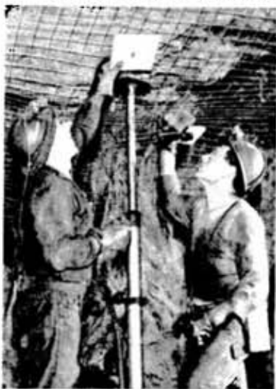
Creighton stope leader Karl Neuman and his partner Roly Boisvenue use the recently developed screenjack to force the screen into the contours of the back for bolting.
