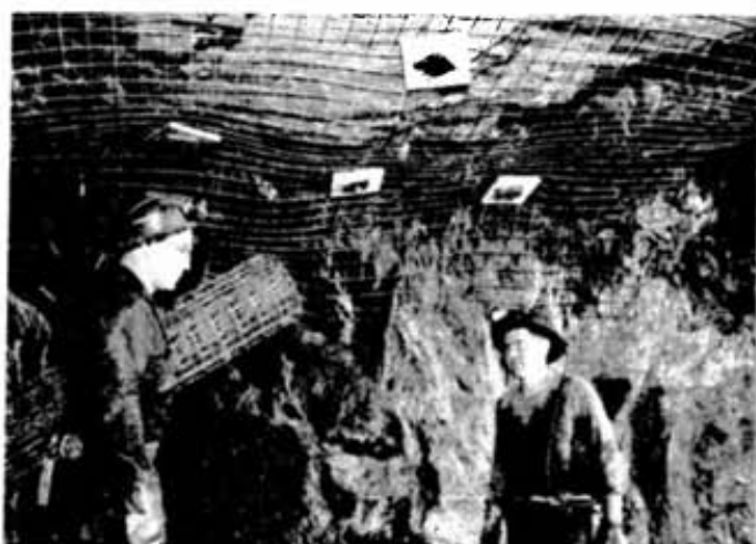
At Frood the welded screen mesh is cut to the required lengths on surface, loaded onto timber trucks as pictured here, and sent underground. The rolls must be of a size to pass through the standard size stope steel chute. Surface switchman coupling the train is Norman Dupuis.
