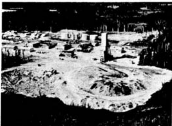
TEMPORARY PLANT. An aerial view of the temporary headframe and sinking plant at the development shaft of Thompson mine. Buildings include hoist room, changehouse, shops, warehouse. The production shaft can be seen in the distance.
