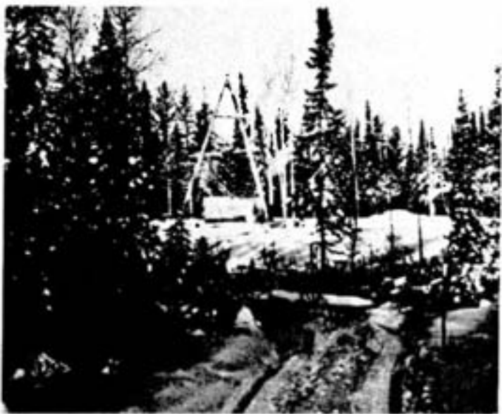
DRILLING. Here is another of the earliest pictures at Thompson, showing a diamond drill testing a rock structure at the proposed location of the first shaft. The thick bush is mostly black spruce.
