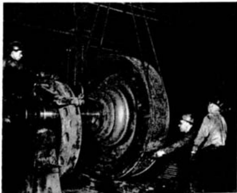
Out for a cleaning and rewinding job, this 6-ton rotor is being returned to the stator of no. 3 blower at Copper Cliff sub-station. On the left foreman Jack Beaudry keeps a close watch as Armand Roy, Bill Bryant and Fern Daigle deftly handle the load.
