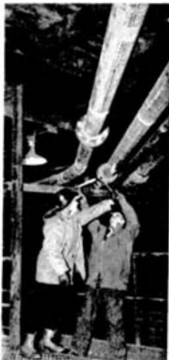
Alex Salo and Al Harris of Jock Rennie's gang give a final check to the flanges on three new 5-inch lines their gang have just installed. Pulverized coal will now travel this route from the coal plant to the reverb furnaces. Pipe work of all kinds is a regular diet for this gang.
