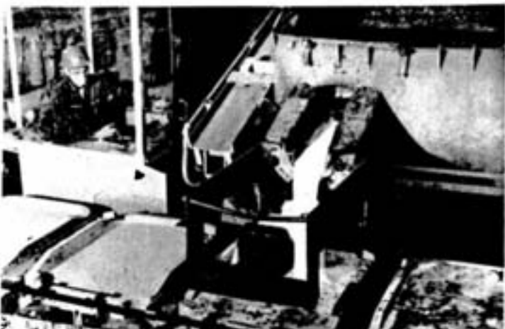
In the top photograph Leo Bremner is shown operating the box crane, lifting anodes from one of the big annealing boxes for shipment to the tankhouse in the refinery. Below is a closeup of the ladle car as it pours a 475-lb. anode into one of the row of moulds. The ladle holds 4 tons of molten bessemer matte, which is poured onto an attached diffuser to spread it over the mould. The operator shown is Emile Romain.
